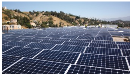
In addition to the high-efficiency E-327 SunPower solar panels, the Forever 21 project involved 19,500 PermaCity Solar Straps and 141 ABB 1,000-volt string-level inverters.
